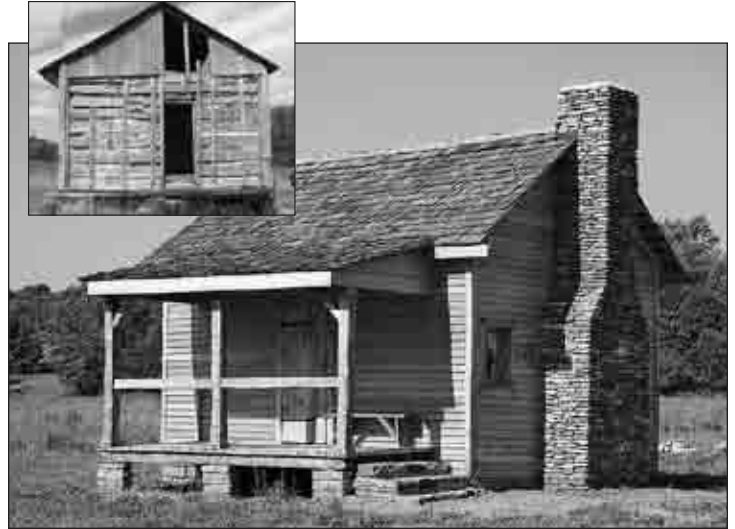
The Edward's family cabin was restored from a crumbling shell (inset) to a close approximation of the cabin used as Price's headquarters during the battle.
